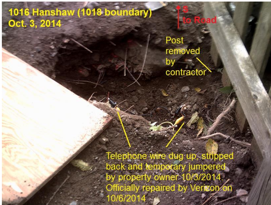
12 conductor cable cut by contractor
